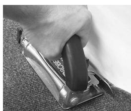
4. Using the guide bar, tuck the carpet into the gully to complete the job. The large handle will permit you to use both hands when necessary.
